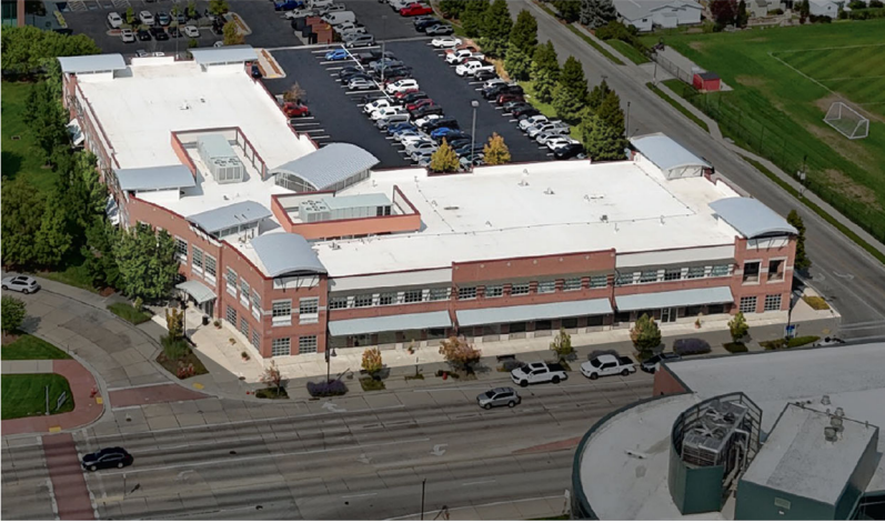
Arbor Plaza Office Building
