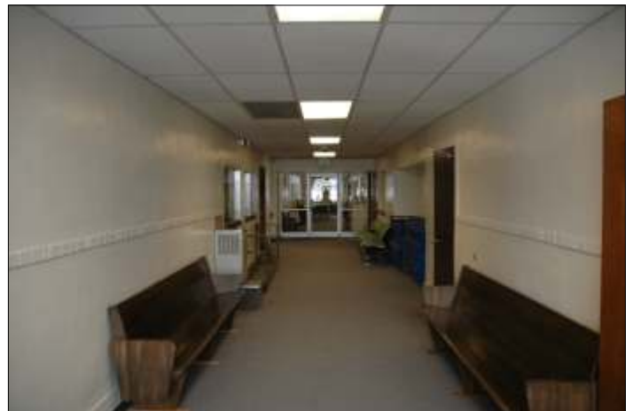
Carpet has been laid over the original floor finish in most classrooms and the corridors (top, above). A suspended acoustical tile system obscures the original tall ceilings.
