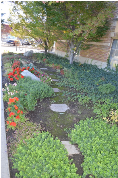
Images 9 & 10: The front landscape has been updated. The planted area adjacent to the building was noted to be very moist, which may be of concern in relation to the foundation of the building.
