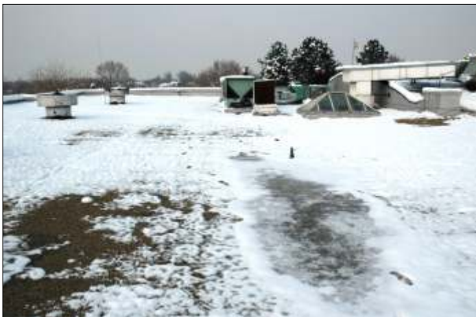
Areas of pooled water indicating insufficient slope toward the roof drains on the west classroom wing. Original gravity globe vents are no longer necessary and can be removed.
