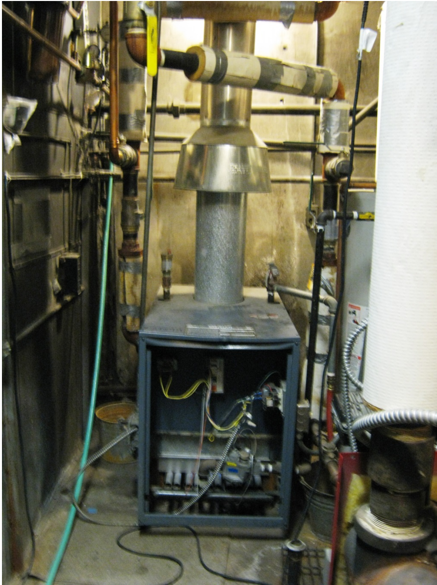
Images 13: The steam boiler was decommissioned and a new furnace installed.
