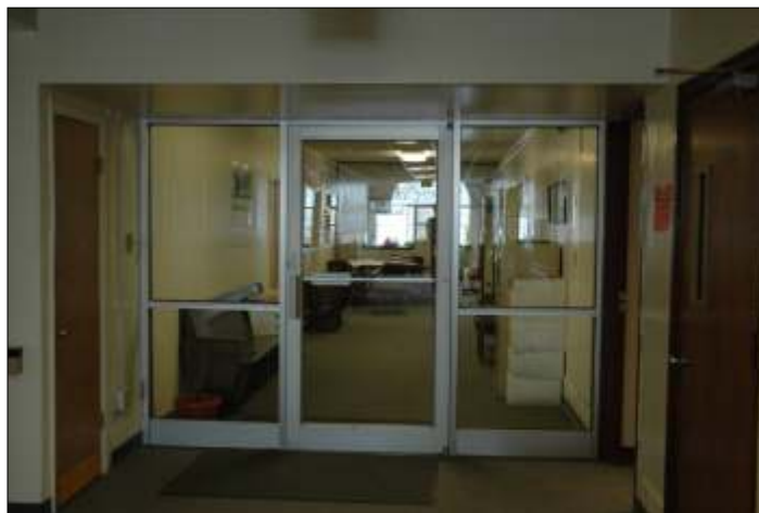
Modern wood slab doors have replaced the original wood panel doors throughout the building. Additional aluminum frame storefront doors have been added to cordon off the south end of the Level 4 corridor.
