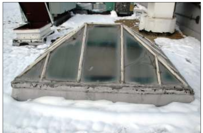
One original hipped-roof skylight remains over the north stairwell but is in poor condition. Replacement skylights over both stairwells are recommended for natural daylight.
