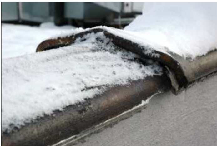
Although the mortar is deteriorating, terra cotta parapet tiles on the north wall of the gymnasium wing are themselves in fair condition.
