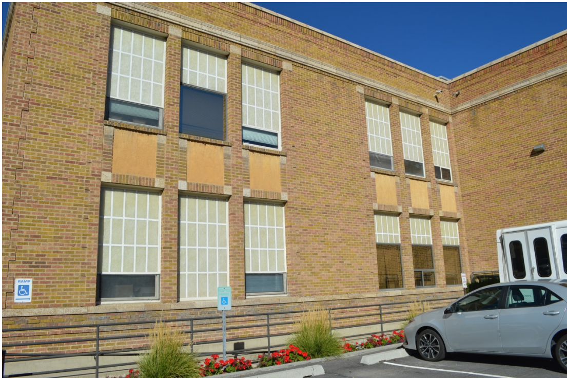
Images 4 & 5: The fiberglass covering on the windows is beginning to degrade, traps moisture leading to mildew, and also blocks the full beauty of the original windows.
