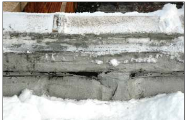
Roofing membranes currently extend up the parapets to terminate just below the coping.
