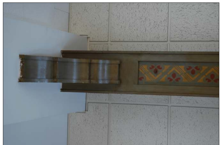
Decoratively painted soffits are below each bow truss of the gymnasium ceiling.
