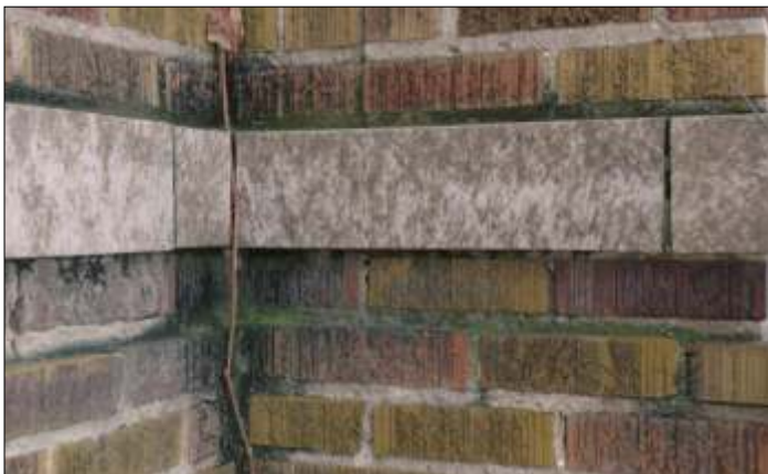
There is some evidence of fungal and microbial growth on the bricks and mortar that should be cleaned by a contractor that specializes in historic masonry buildings.
