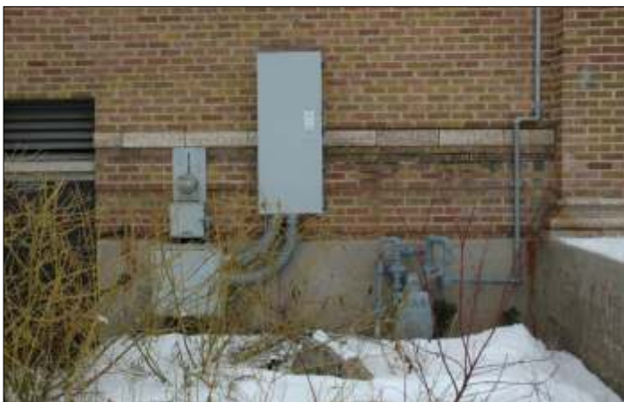
The concrete foundation is in good condition, with no substantial deterioration of the plaster finish.
