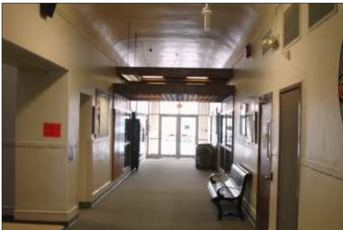
The central corridor on Level 2 retains its original high coved ceiling. With the exception of the gymnasium the remainder of the corridors and rooms have dropped ceilings in place.
