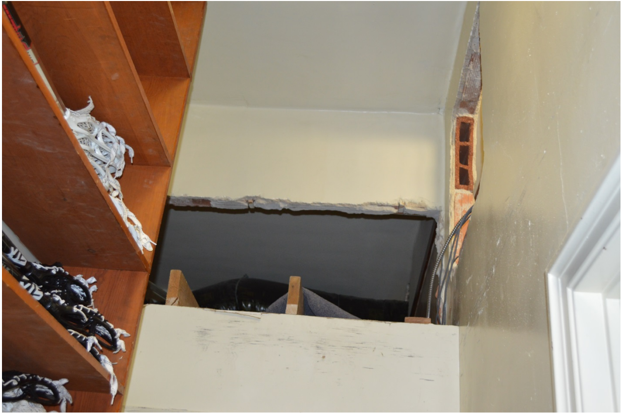
Image 3: The of the soft clay tiles of the interior wall structure is visible where holes have been made to run mechanical/electrical systems.
