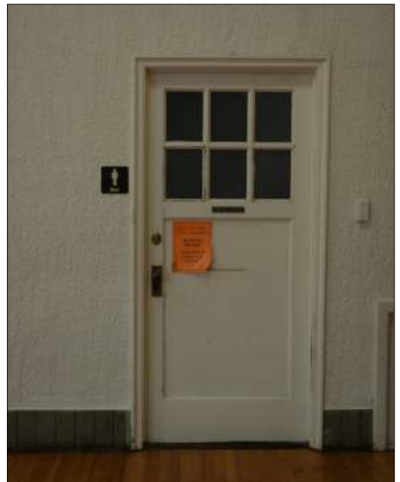
The original wood panel doors with a divided glass upper panel still remain at the entrances to the stairwells that lead from the gymnasium to the restrooms below.
