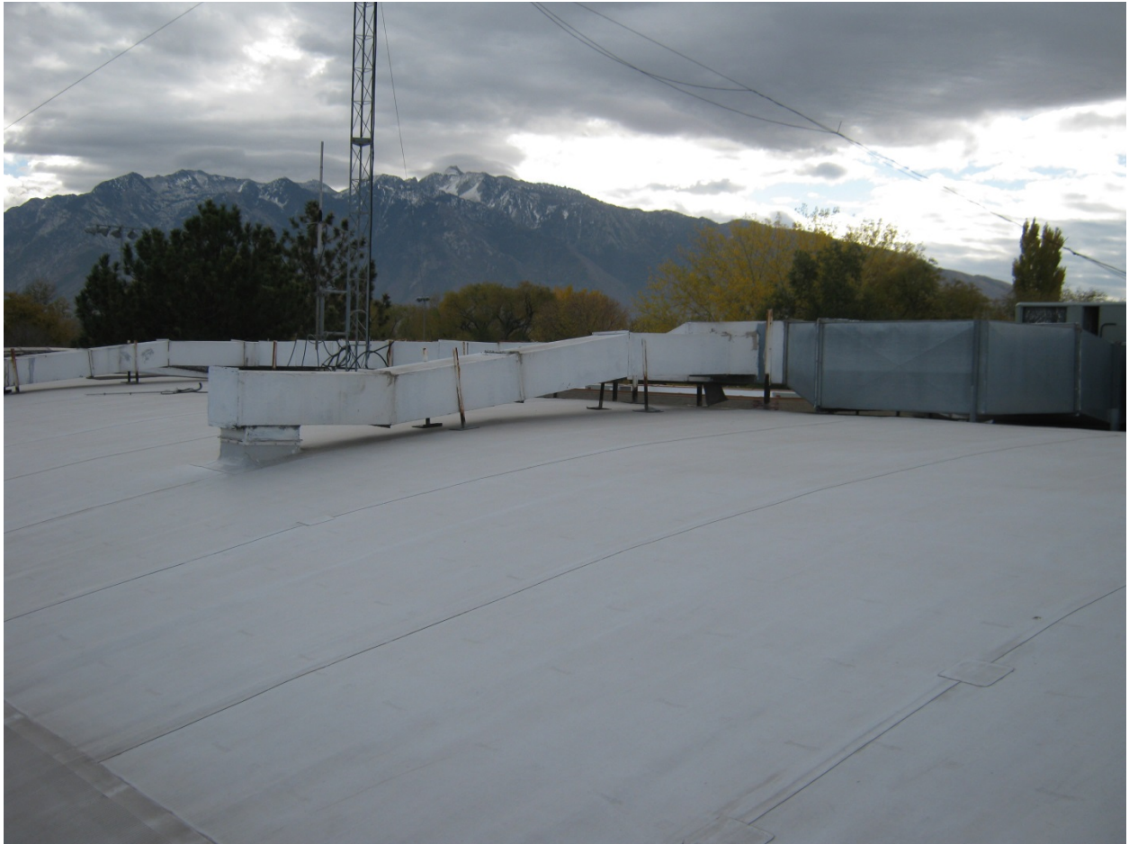
Images 11: The roof membrane on the gymnasium wing is still in good condition.
