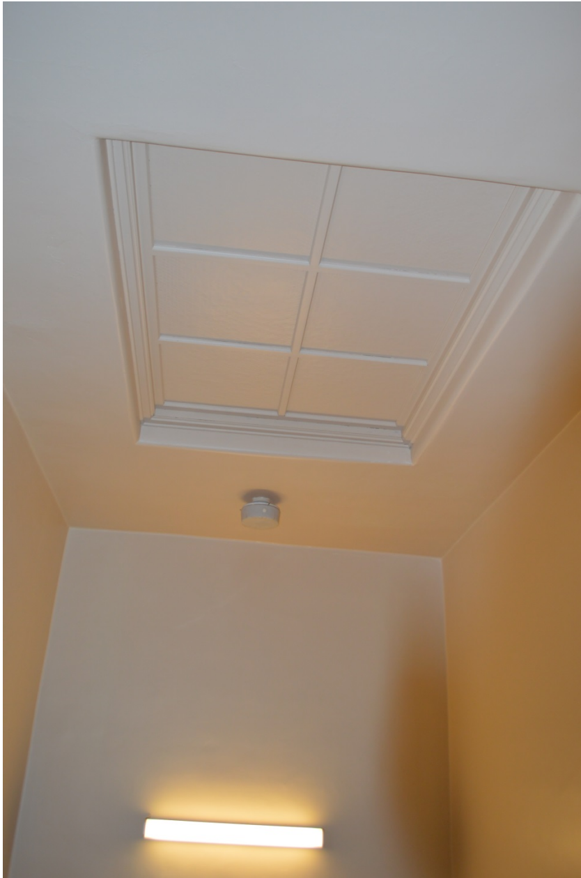
Images 12: The interior glass of the skylight has been painted over, for aesthetic purposes (the skylight is in need of repair/replacement).
