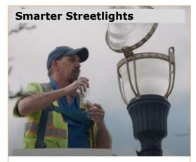
In 2019, Sandy City started converting streetlights from high-pressure sodium (HPS) bulbs to high-efficient light-emitting diode (LED). Each LED fixture uses about 70% less electricity than HPS lamps, reducing operating costs, energy use and air pollution emissions.
