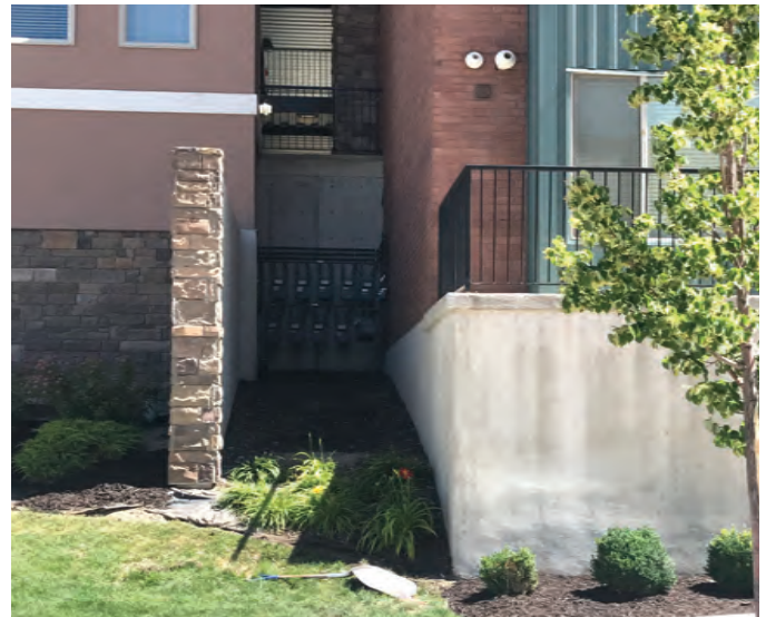
Figure 1104 - Wall mounted equipment screened with a masonry wall
