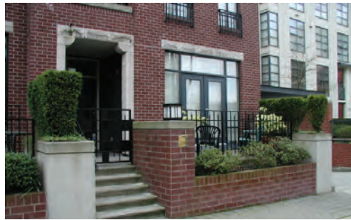
Figure 509 - High-quality materials on residential buildings
