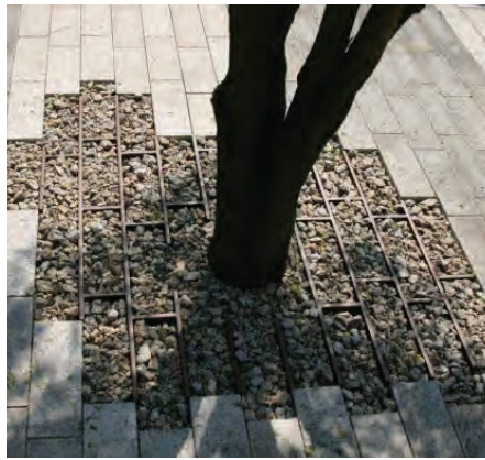
Figure 701 - Brick cut-out tree grate
