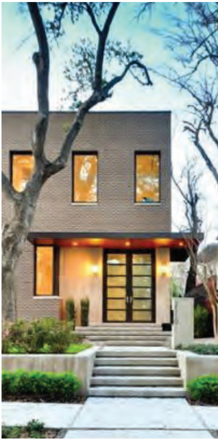
Figure 506 - Residential entrance located above the sidewalk grade
