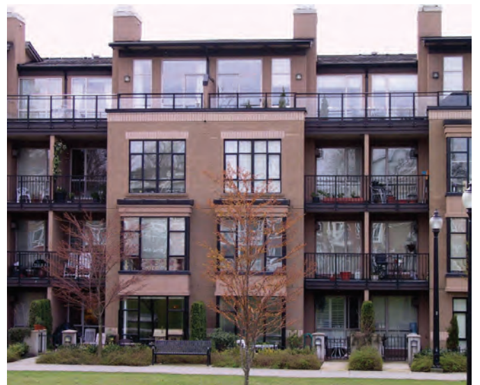
Figure 407 - Example of a building with a prominent top section
