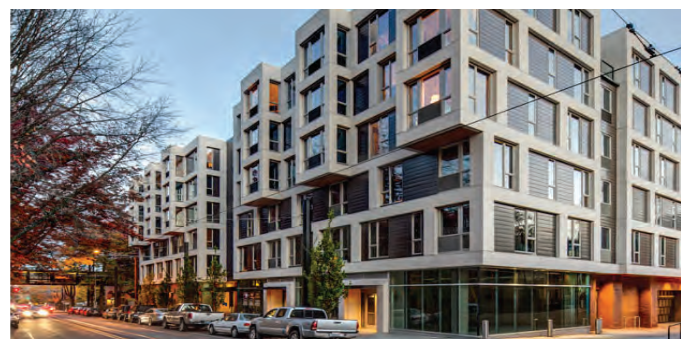
Figure 505 - Recessed corner treatment and a mix of architectural material
