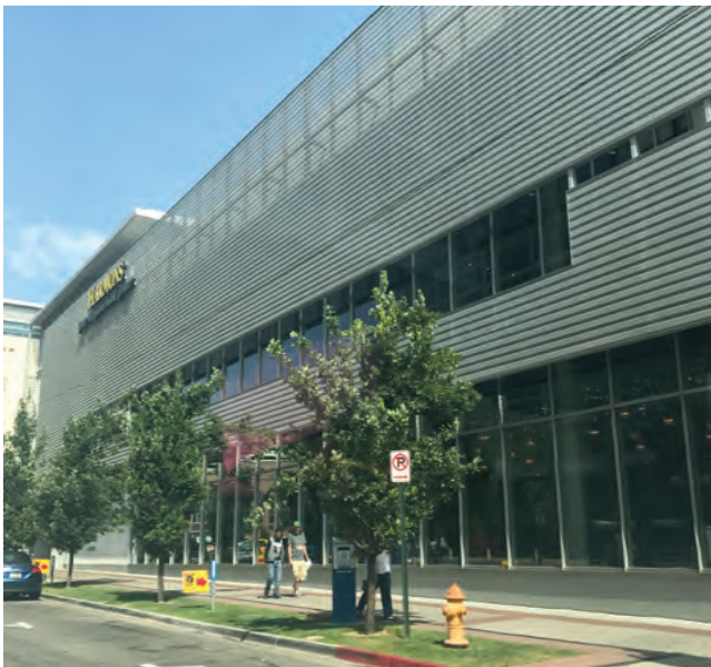
Figure 607 - Parking garage screened as an architectural element
