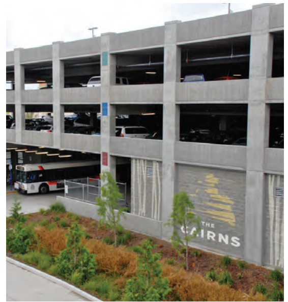
Figure 606 - Parking garage decorated to brand The Cairns
