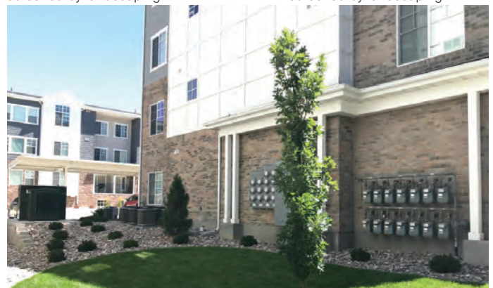
Figure 1107 - Wall mounted equipment hidden from pedestrian realm
