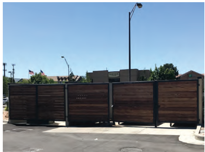
Figure 1103 - Dumpsters enclosed using high quality materials
