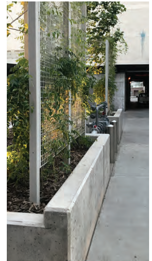
Figure 1106 - Utility boxes screened by landscaping
