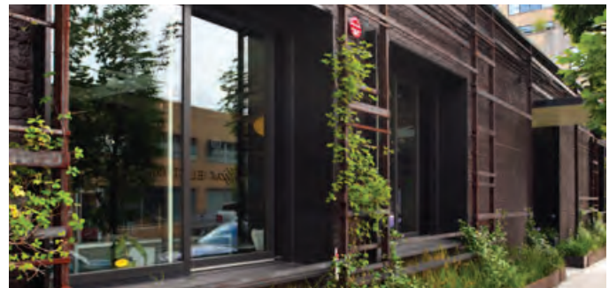
Figure 504 - High-quality materials on a building frontage
