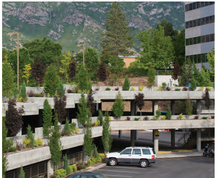
Figure 608 - Parking garage left open with native landscaping
