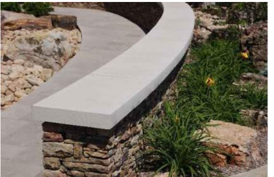
FIGURE TWO SEAT WALL CONCRETE CAP MATERIALS
