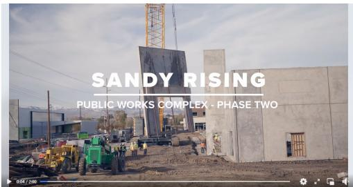
The walls are rising over at our Public Works complex, where phase two construction is well underway. These concrete slabs weigh up to 170,000 pounds and are carefull...
