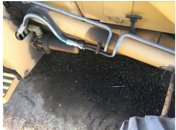
Photo #12 Soil staining of hydraulic fluid from the backhoe.
