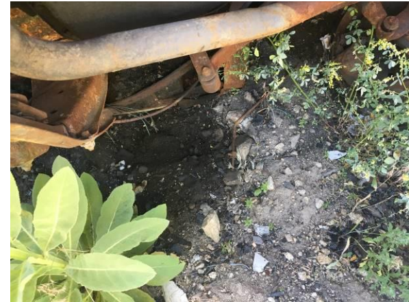
Photo #24 Stained soil under the vehicle in the area of the fire.
