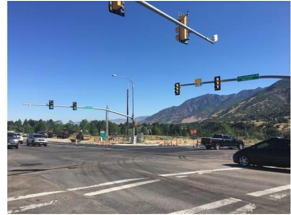
Photo #36 North-adjointing intersection at Wasatch Blvd and Little Cottonwood Canyon.
