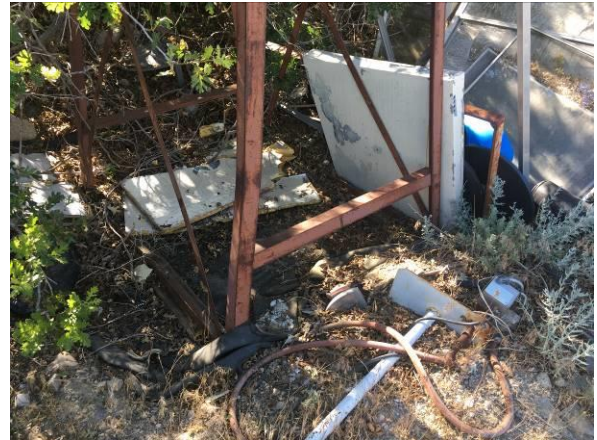
Photo #26 A plastic liner was observed beneath the tank. No staining was observed.
