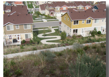
Secondary/Neighborhood Access at Quarry Bend
