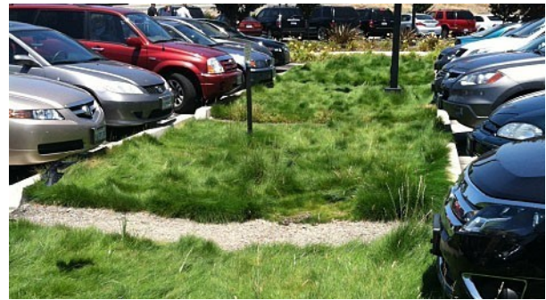
Vegetated swales, such as this installed in a parking lot, can both treat and convey runoff, eliminating the need for some catch basins and pipes.
