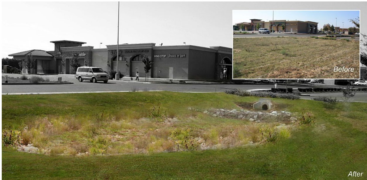
Basins that are thoughtfully designed and planted can manage stormwater from a larger area, while still offering aesthetic appeal.
