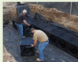
Cudo Cubes are an example of a typical modular block system.
