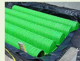
Triton stormwater chambers are a typical semi-circular linked chamber system.
