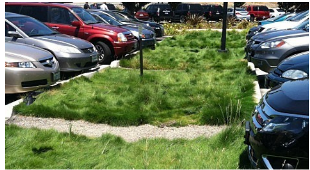
Vegetated swales, such as this installed in a parking lot, can both treat and convey runoff, eliminating the need for some catch basins and pipes.
