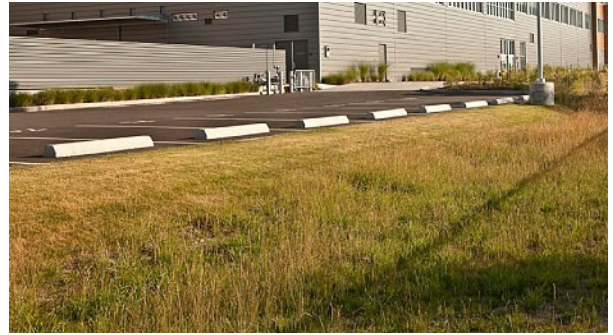
Filter strips can be as simple as a gentle slope covered in grass that receives runoff from an adjacent strip of parking stalls.
