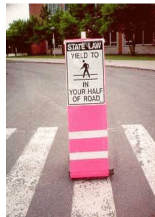
Figure 10. Regulatory pedestrian crossing sign in New York State.
