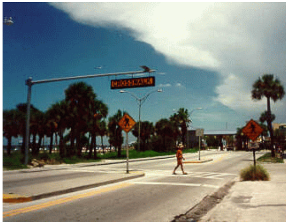
Figure 7. Overhead crosswalk sign in Clearwater, FL.
