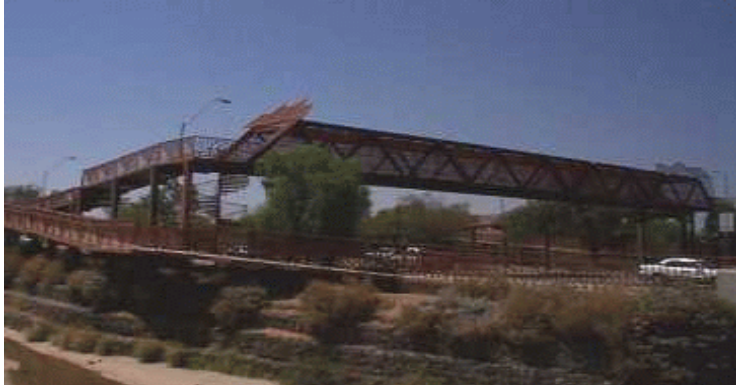
Figure 38. Grade-separated crossings sometimes are used when other measures are not feasible to provide safe pedestrian crossings.
