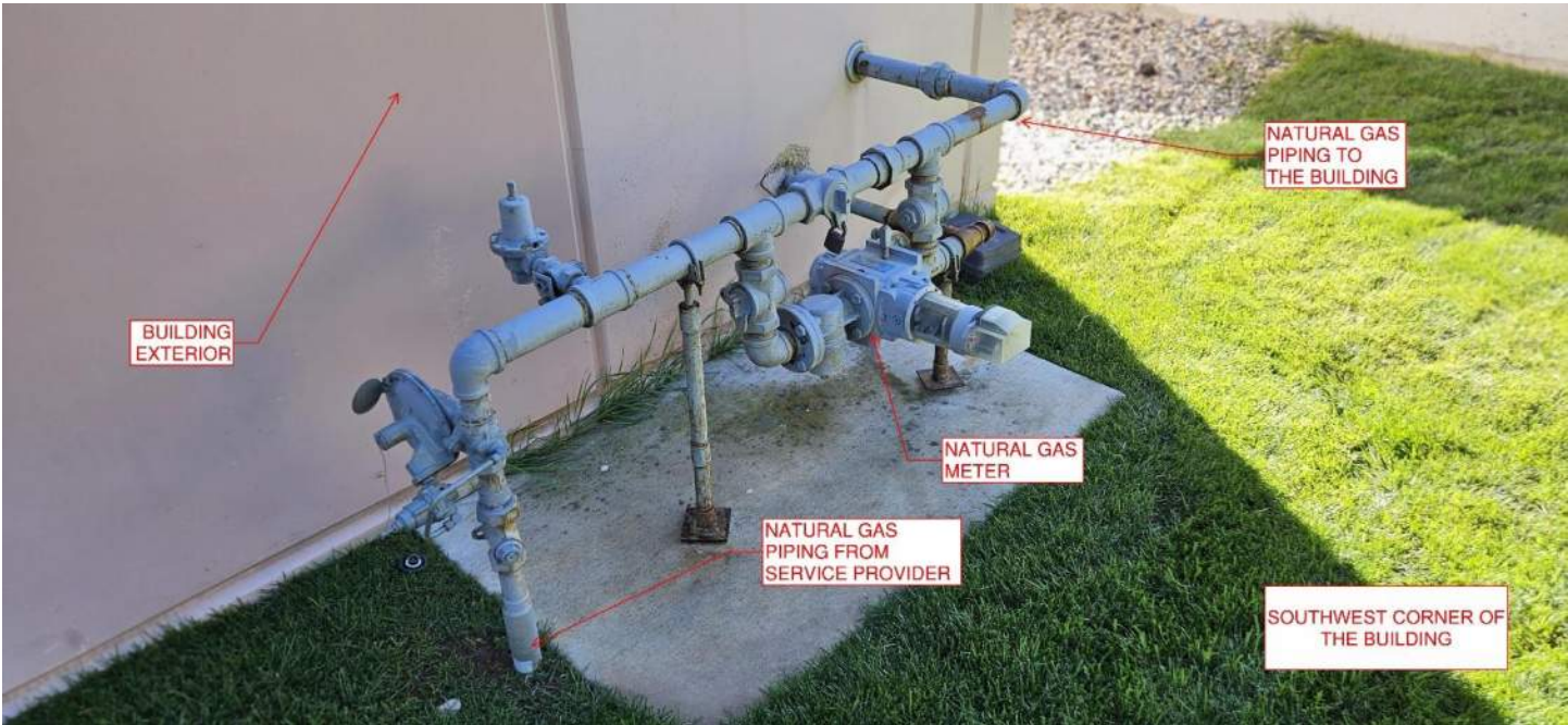
FIGURE 19 - NATURAL GAS SUPPLY METER
