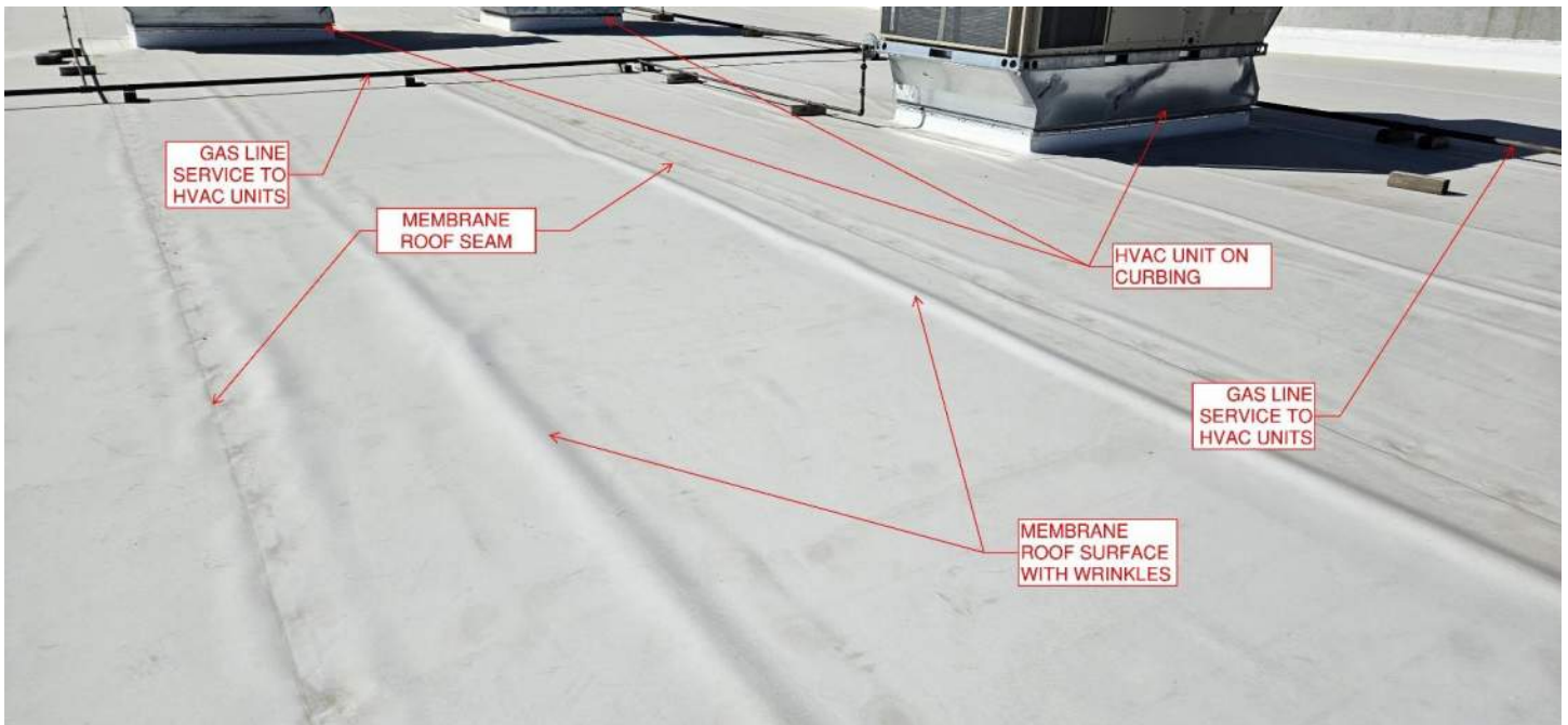
FIGURE 26 - MEMBRANE ROOF
