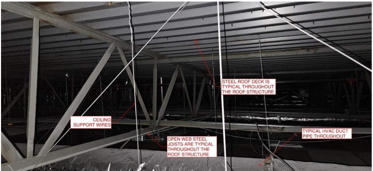
FIGURE 7 - ROOF FRAMING
