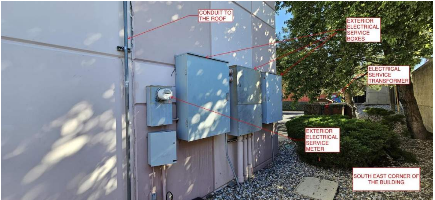
FIGURE 23 - ELECTRICAL SERVICE PANELS
