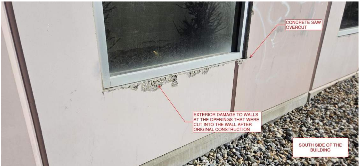
FIGURE 20 - CHIPPING AT SOUTH WINDOW SAWCUTS
