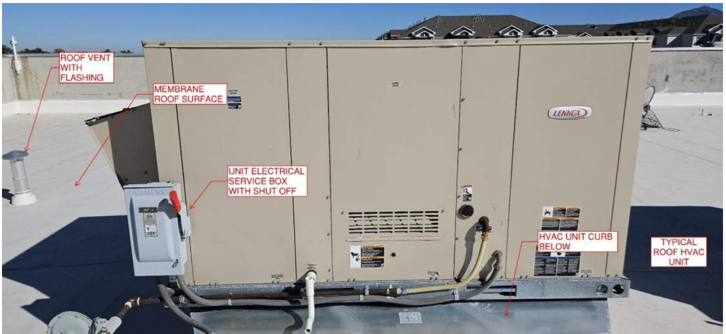
FIGURE 24 - HVAC ROOFTOP UNIT
