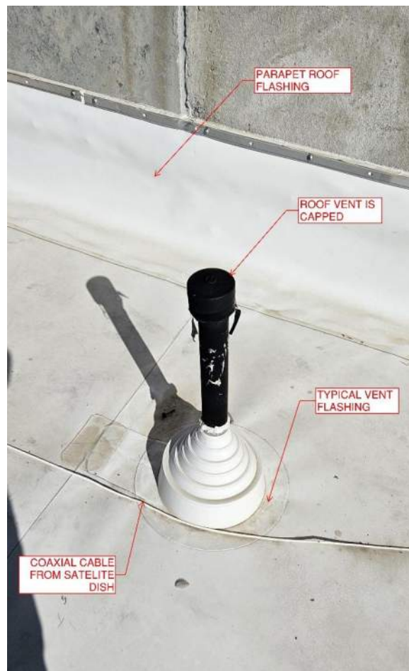
FIGURE 32 - CAPPED ROOF VENT WITH TYPICAL FLASHING
