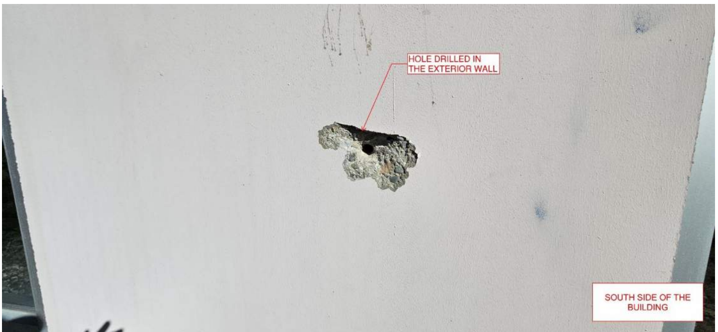
FIGURE 21 - WALL PENETRATION AT IN THE SOUTH WALL
