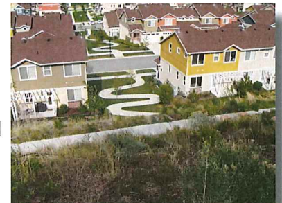
Secondary/Neighborhood Access at Quarry Bend
