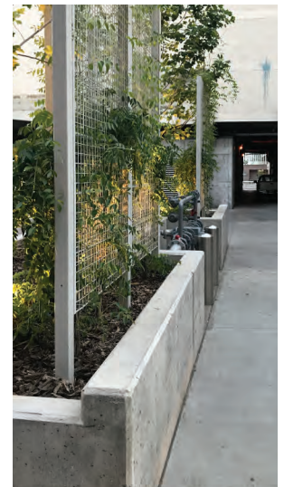
Figure 1106 - Utility boxes screened by landscaping
