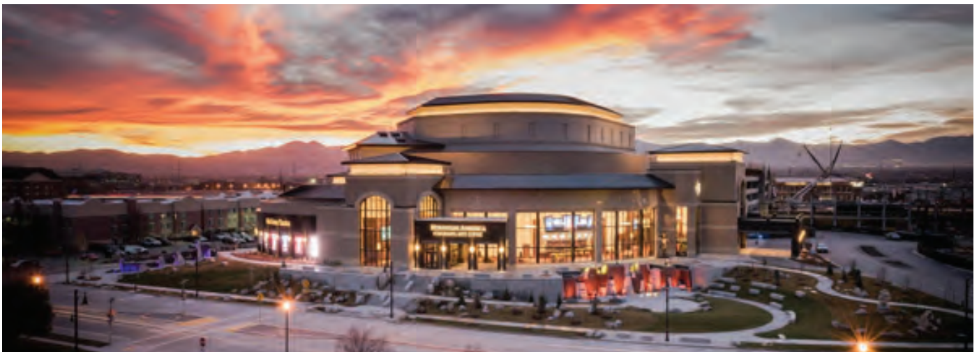
Figure 515 - Hale Centre Theatre with high-quality materials and design
