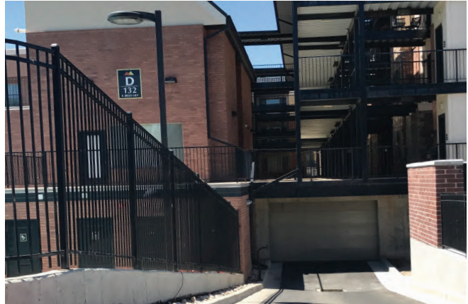
Figure 1101 - Loading area screened with a masonry wall
