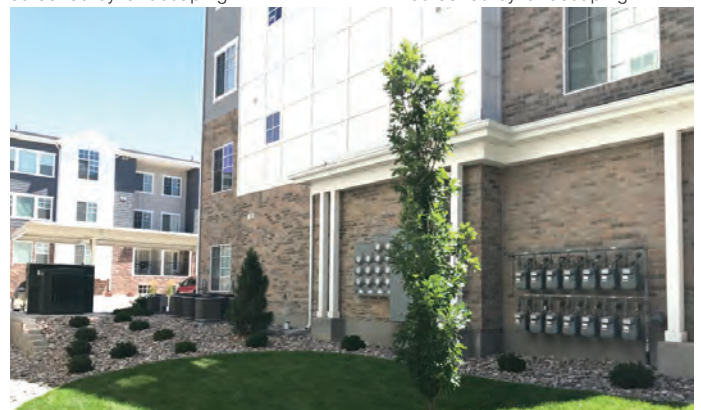
Figure 1107 - Wall mounted equipment hidden from pedestrian realm
