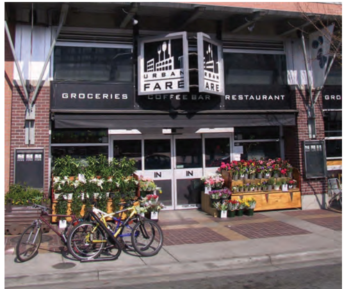
Figure 220 - Outdoor Displays as a right of way encroachment
