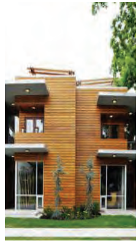
Figure 522 - Architectural roof capping
