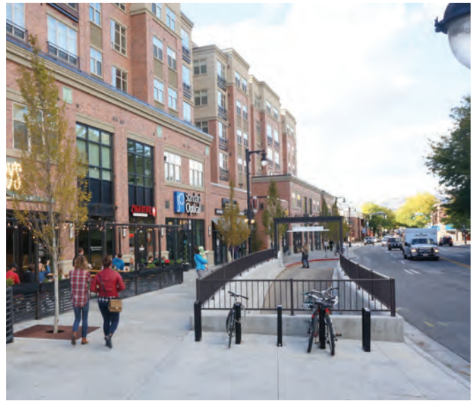
Figure 611 - Parking entrance blends with the streetscape
