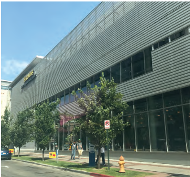
Figure 607 - Parking garage screened as an architectural element
