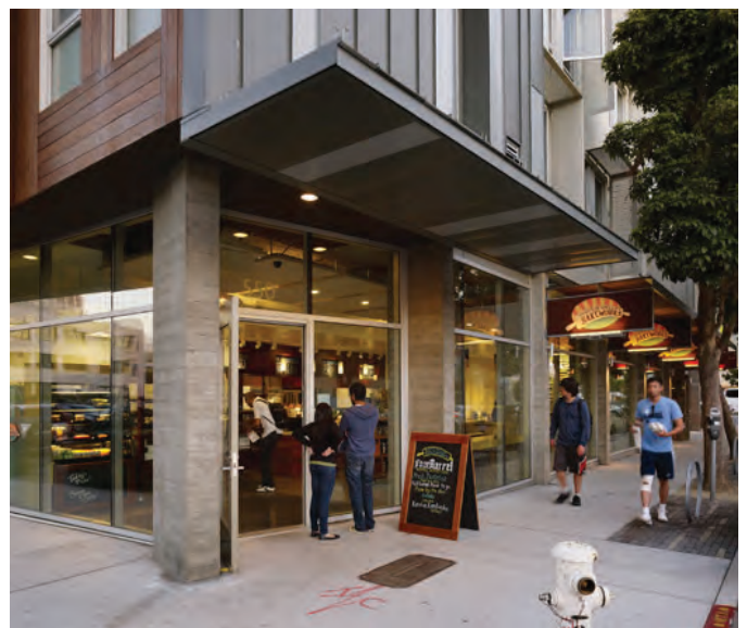
Figure 221 -Outdoor Signage as a right of way encroachment
