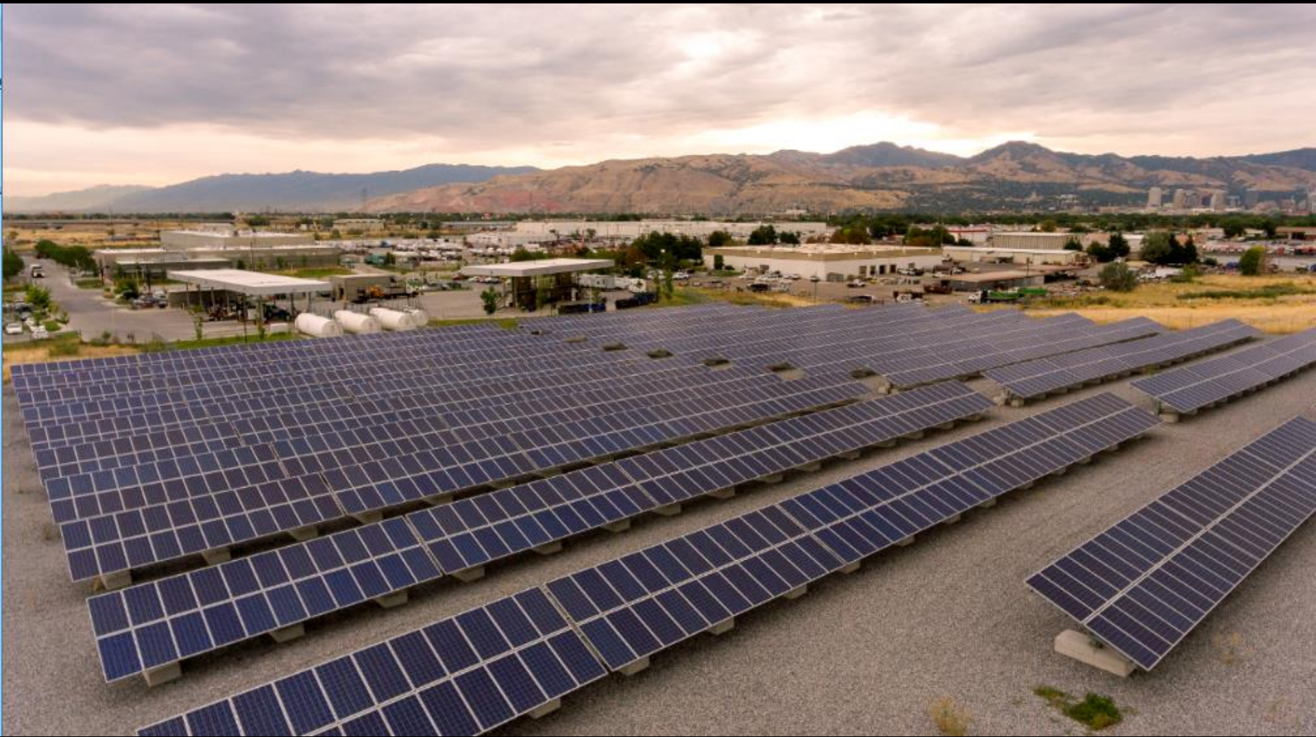
Salt Lake City Solar Farm | Old Landfill Site
