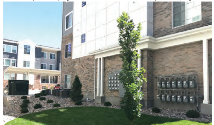
Figure 1107 - Wall mounted equipment hidden from pedestrian realm
