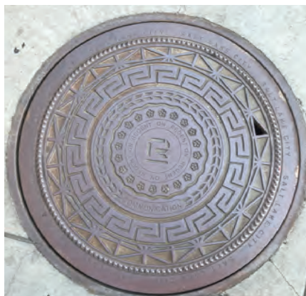
Figure 707 - Local example of a branded manhole cover
