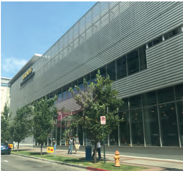
Figure 607 - Parking garage screened as an architectural element
