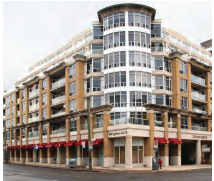
Figure 406 - Example of a building with a strong base, middle, and top
