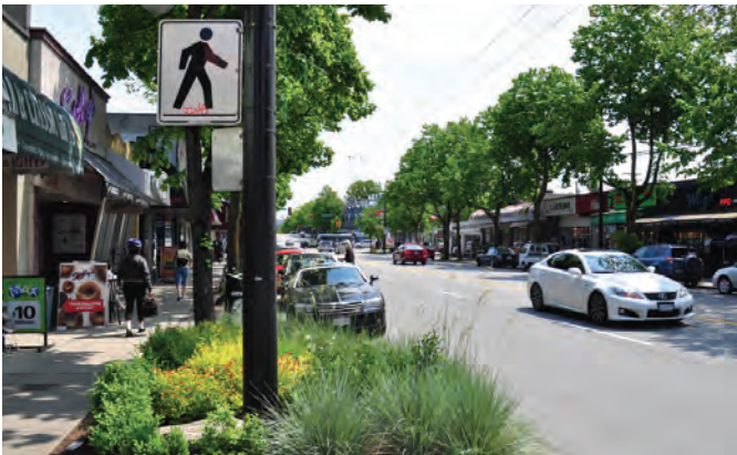
Figure 206 - Parkstrip used to soften the street edge
