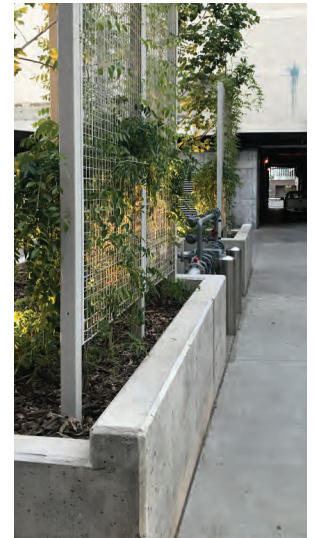
Figure 1106 - Utility boxes screened by landscaping
