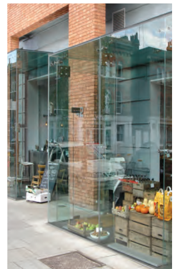
Figure 503 - Protruding display windows for fenestration
