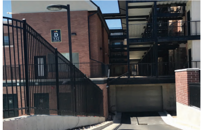
Figure 1101 - Loading area screened with a masonry wall
