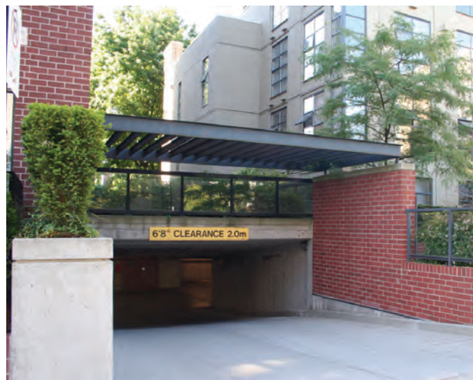
Figure 613 - Parking entrance architecturally enhanced with brick and awning
