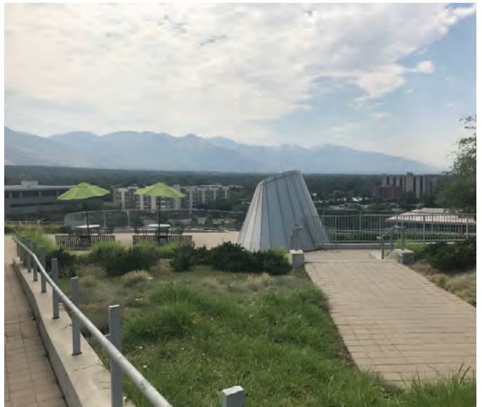
Figure 1004 - Landscaped green roof
