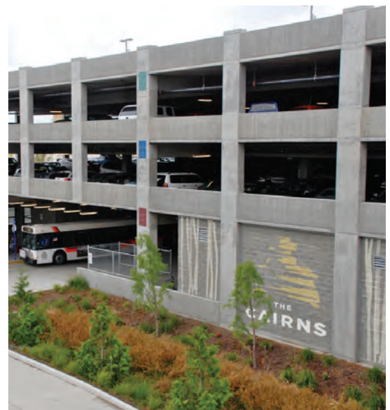
Figure 606 - Parking garage decorated to brand The Cairns
