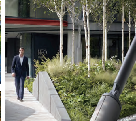
Figure 743 - Border along in-grade planter for safety
