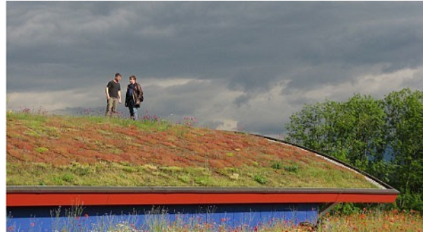
Green roofs are unique stormwater features which also provide a variety of diverse benefits to building systems as well as inhabitants and users.
