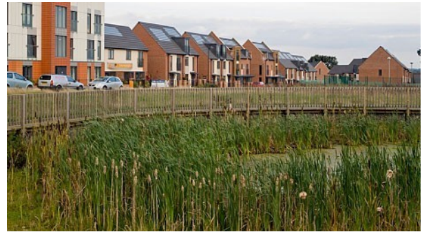
Though more technically complex, constructed wetlands have the potential to provide the most water quality improvements of any naturalized system.
