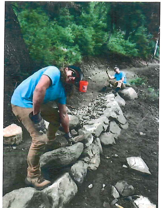
Building a retaining wall at Cardiff Fork
