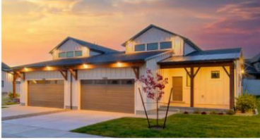
Mixing middle housing examples at the Richard Dawkins
