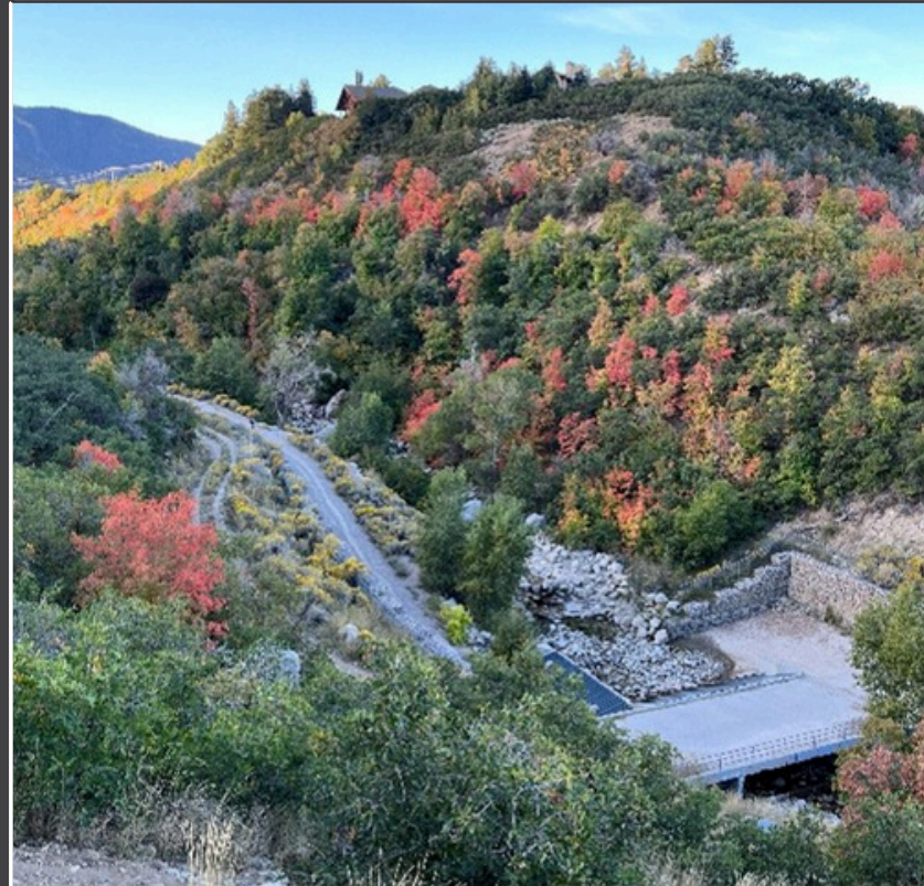
Raw Water LITTLE COTTONWOOD CONDUIT Placed in service 1931
