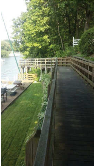
Elevated Multi-use Trail
