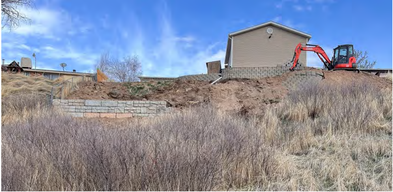
March 2025 Site Photo
