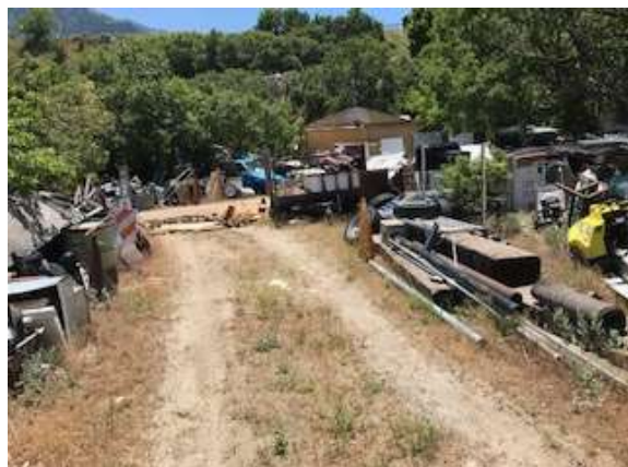
Debris on Subject
