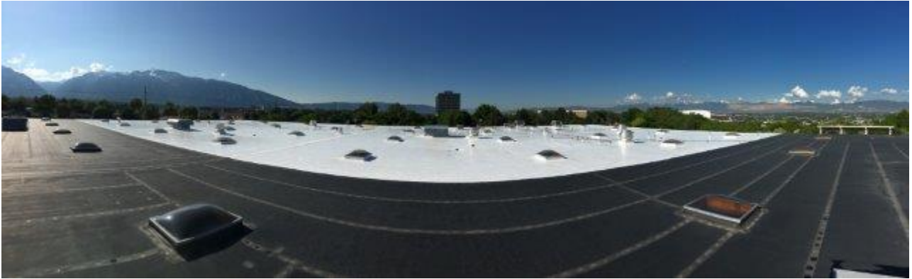
Roof replacement project at Public Operations - 9150 S 150 E
