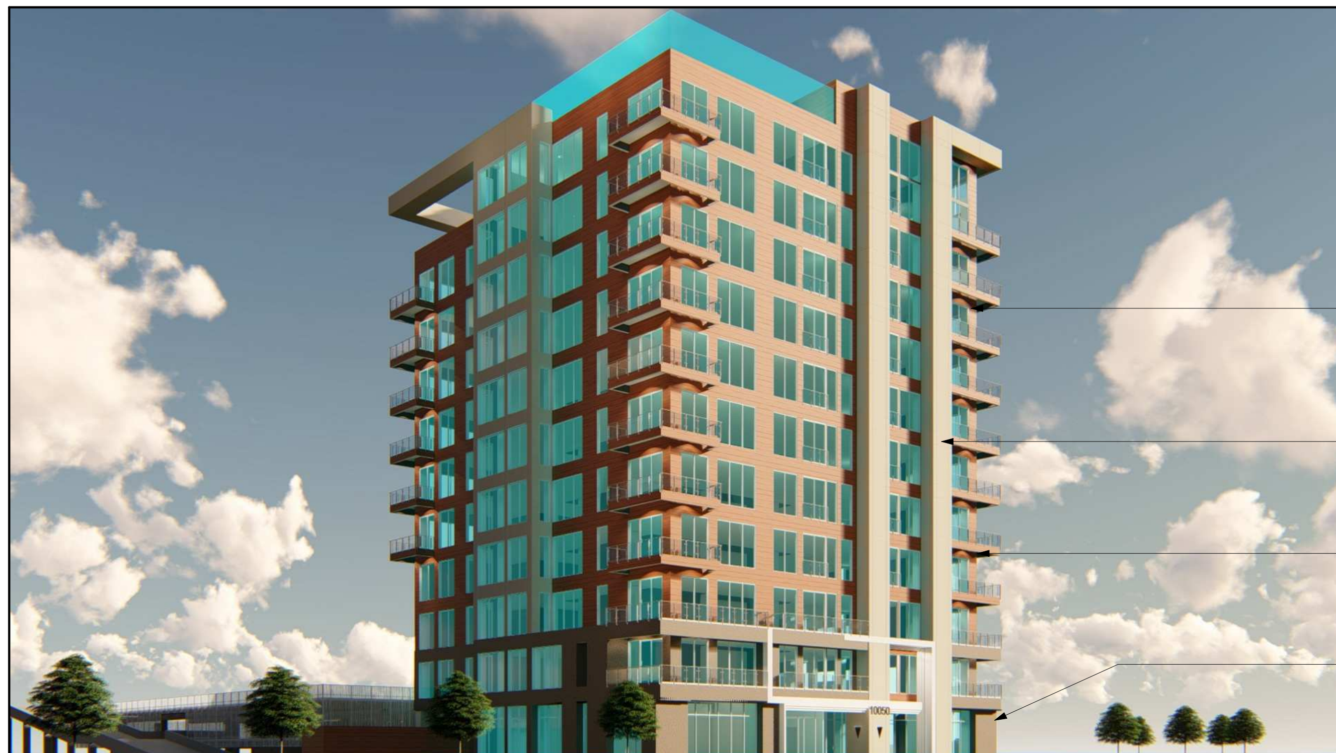
NORTH WEST VIEW
