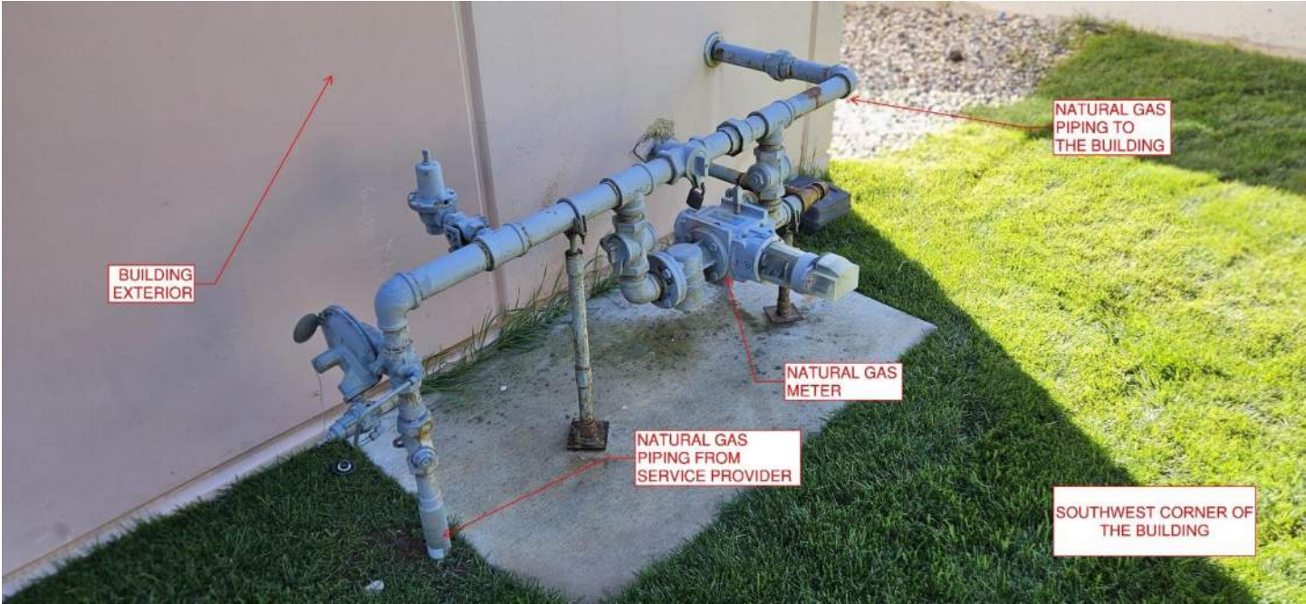
FIGURE 19 - NATURAL GAS SUPPLY METER
