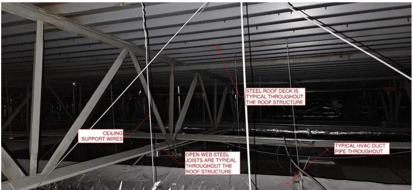
FIGURE 7 - ROOF FRAMING
