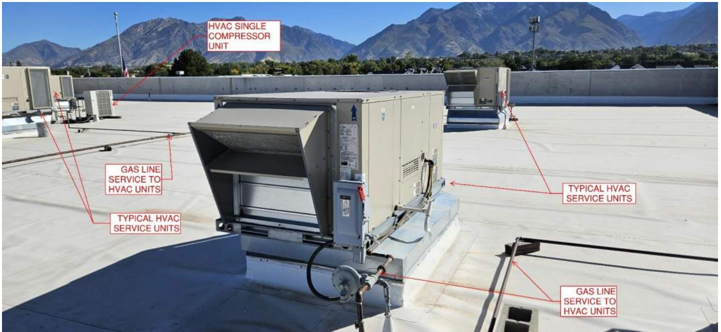
FIGURE 28 - MULTIPLE ROOFTOP HVAC UNITS
